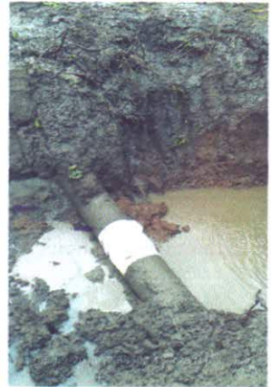
FIGURE: 3 REPAIR WORK
