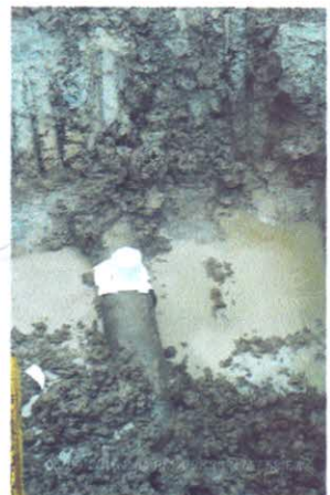
FIGURE: 3 REPAIR WORK
